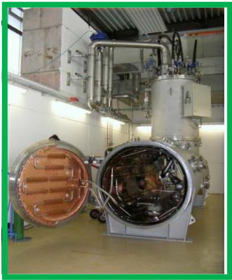
HOBICAT, BESSY Operational Bi-Cavity Horizontal Test Facility
